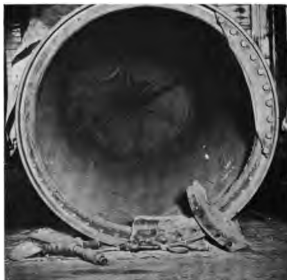
Fig. 4. Steam Cylinder of Flat-Work Ironer which Burst, Wrecking Building.
